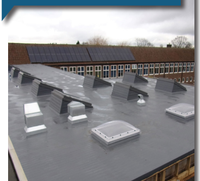
Overview of work from 2016
