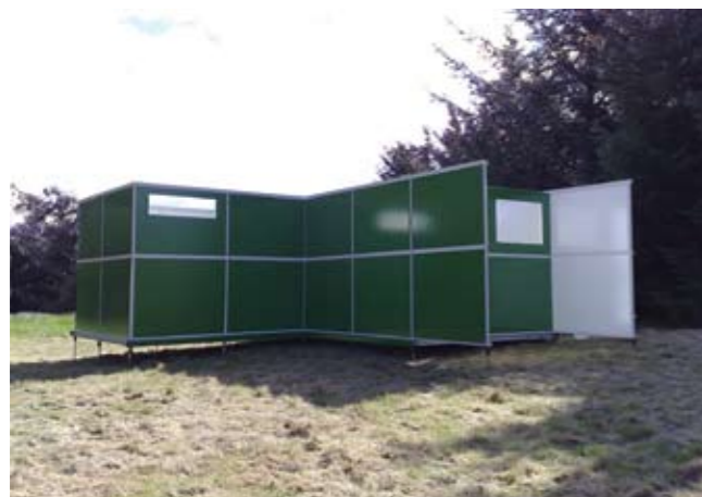
8 The shelter with all of the wall sections completed.
