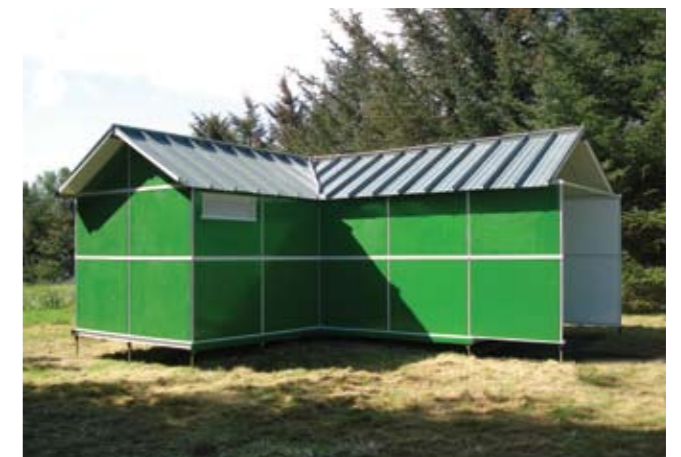
11 The completed shelter with a covered area on the right end elevation.
