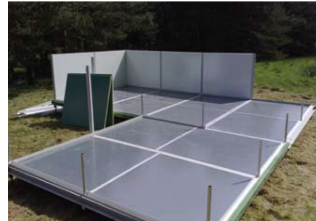
5 The fully insulated wall panels are then slid into position between the tubular cruciform post wall supports. The entrance door can be positioned on either side of the shelter. The windows can be positioned in the walls to suit the users needs.
