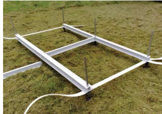
1 No foundations for the shelter are required. The floor beams and the wall plates are used as a guide for positioning the adjustable floor support leg plates. This is a visual process and need not be too exact. The fitting of the wall plates and floor support beams will square everything up.
