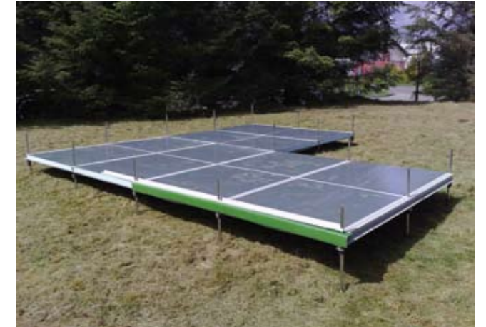
3 When all the floor panels are positioned the base of the shelter will now be rigid. You can now move on to assembling the walls.
