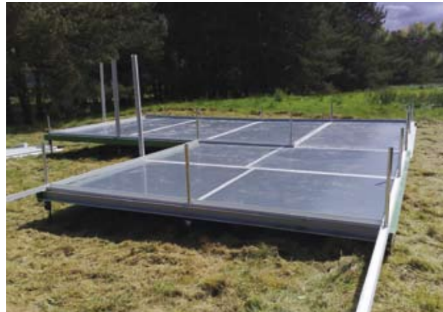
4 The tubular wall supports are slid into position over the upright sections of the floor support plates. These cruciform posts lock into the pre-cut channels of the insulated wall panels.
