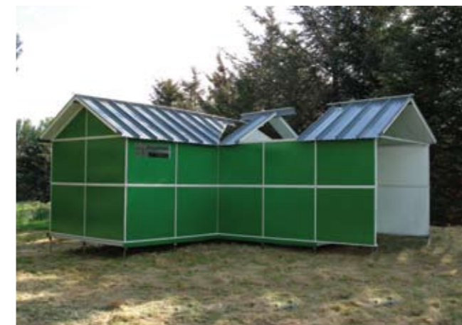
10 The shelter with the roof nearing completion
