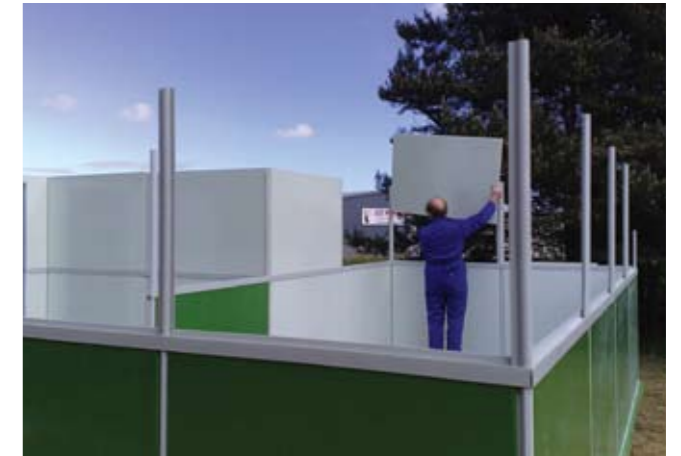
7 Inserting the upper wall panels.
